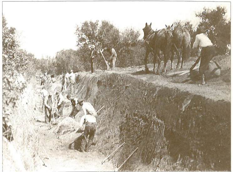
The water district began in 1920 as an irrigation district. Water was delivered to ten acre plots in Citrus Heights via the North Fork Ditch Company, shown being dug here. Hand shovels and "two horsepower" excavators such as the one on the right were the latest in equipment.
