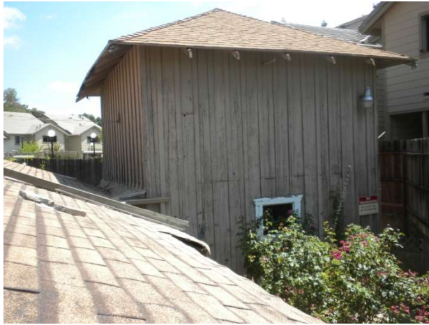
View of the 14 Mile House tank house
